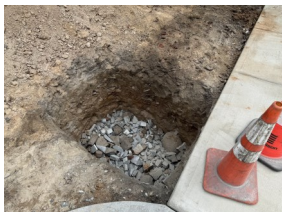
Deep dry wells and gravel enhance yard drainage
